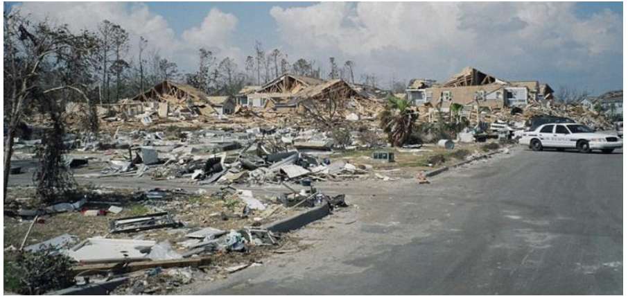
New Orleans after Hurricane Katrina
