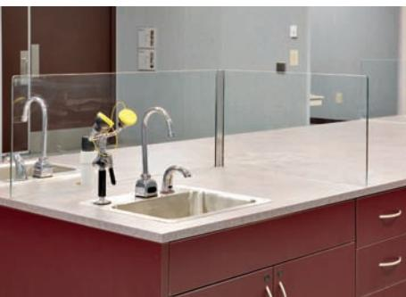
**Clear splash guards are set into the solid surfacing counter and enclose the stainless steel sink.**
