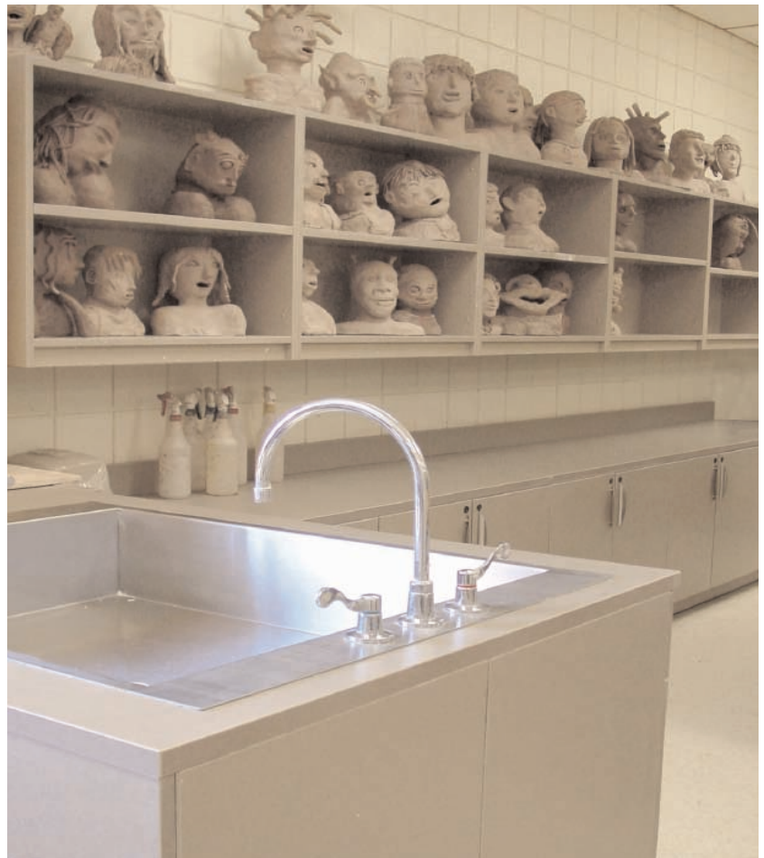
This oversized sink is built into a peninsula island for multiple access by students.
