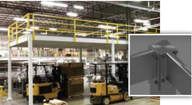
HSS/TUBE STEEL Typically selected when a platform requires closed shapes for washdown and cleanliness.
