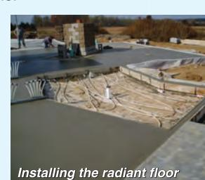
The Mead facility has 8 closed-loop ground-source heat pumps for heating & cooling. There are 4 water-to-water units for multi-zone in-slab hydronic-radiant floor heating, with a 16 ton heating/cooling capacity rating. There are also 4 water-to-air units for multi-zone ventilation & conditioned-air, with a 13 ton heating/cooling capacity rating. Outside the building there are 32 exterior heat-exchange ground loops, each 600' long, buried 8 feet deep.
