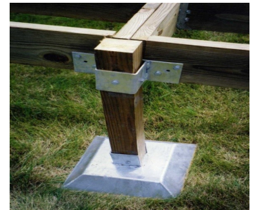
Non-intrusive pan type footing.
