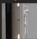
Doors open a full 180 degrees and lift off easily for curatorial convenience. No tools are required.
