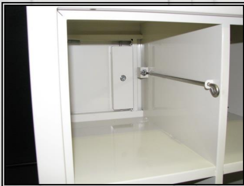
INTERNAL VIEW- LATCH RELEASE
